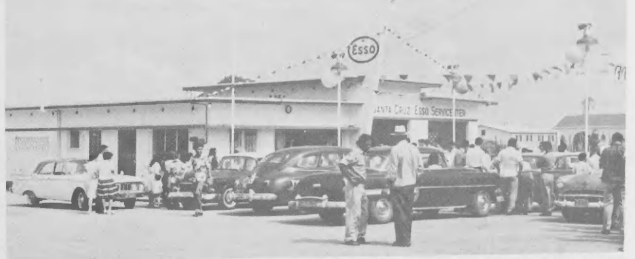
WHEN OWNER Frans Croes turned on the modern, high-speed gasoline pumps, a line of customers awaited attendants. Two 4000-gallon tanks store Esso regular and premium gasolines.
